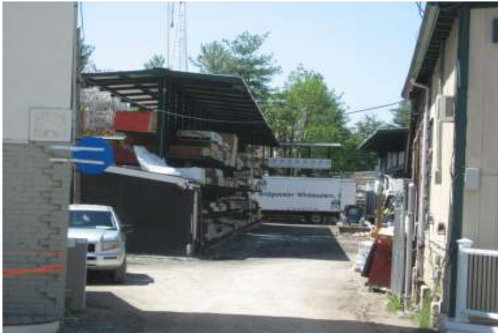
View of storage racks (west aisle) looking south
